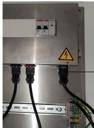
1 Power supply panel connector (X1) at the power distribution box
