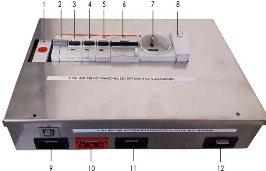
Fig. 15: Power distribution box (figure with options)
