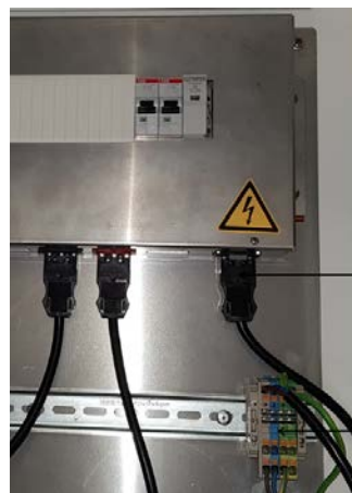
Fig. 20: Terminal block -X0
