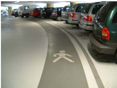
Fig. 1: Safety marking on the road
